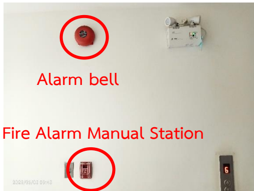
Alarm bell & Fire Alarm Manual Station
